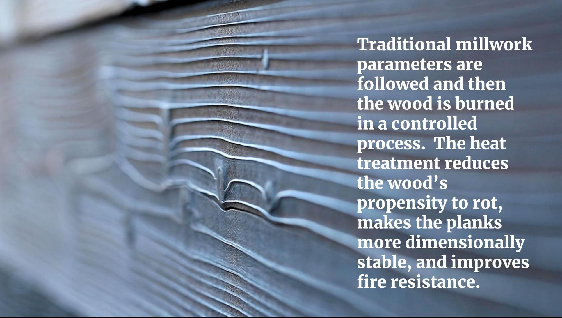
A close-up photograph of a stack of dark, charred wood planks. The planks are stacked horizontally, and the image shows the edges and surfaces of many layers. The wood has a wavy, textured appearance, likely due to the heat treatment process mentioned in the text. The lighting is dramatic, highlighting the grain and the charred texture of the wood. The background is blurred, focusing attention on the texture of the wood.
